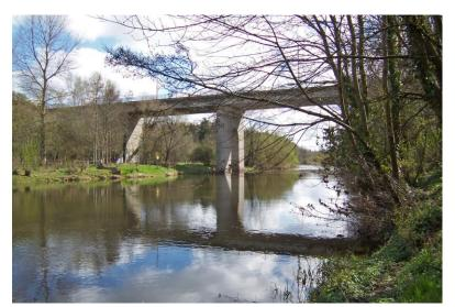
Ossory Bridge brings the Ring Road over the River Nore. It was designed by De Leuw, Chadwick Ó hEocha and opened in 1984. The deck of the bridge is a reinforced concrete slab supported on precast beams. These are mounted on two piers and on abutment walls founded on the rock at either side of the river.
