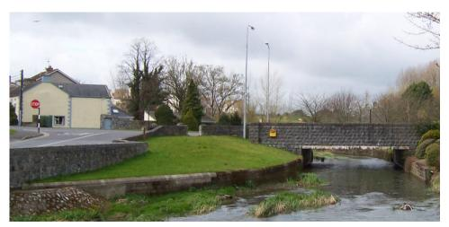
6. Waterbarrack. This modern bridge connects Dominic Street with the Butts Roundabout. It is a reinforced concrete slab laid on piers.
