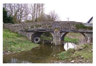
7. This hump-backed two-arch bridge is on the road to Ballycallan and Kilmanagh. In recent years, it has been found necessary to put a traffic light on both ends of the stretch of road crossing the bridge, because cars and lorries have been using the Circular Road and this bridge to bypass Stephen Street and Dominic Street. On the right you can see damage done to the parapet of the bridge.
