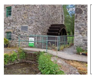
At the end of the mill pond is a channel leading to the mill wheel. The grid over the entrance to this channel is there to prevent dirt and branches, which are carried down by the river, from getting into the millrace. They might damage the mill wheel or stop it. This wheel is in working condition and visitors to the mill can see it in action during the summer. Mullins Mill is open to the public.
