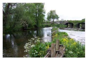
This weir on the King's River or Avonree is at Kells, County Kilkenny. The millpond is on the right. This provides a supply of water to turn the millwheel. Water from the millpond can be seen spilling over the weir, into the river, which is at a lower level than the pond.
