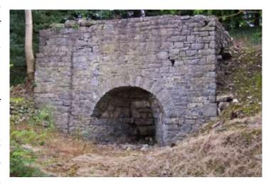
Up on top there was an open pot where layers of fuel, usually coal and layers of limestone were placed on top of one another. The kiln was then set on fire and burned for several days. The very high temperatures in the kiln converted the limestone into quicklime and this was raked out from the bottom of the kiln. It had to be handled very carefully as it was caustic – in other words it could burn the bare skin. It had to
