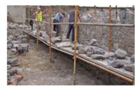
You can get some idea of how stone walls were built long ago, by looking at the way these three men are constructing a stone garden wall at the back of Rothe House in Kilkenny.
