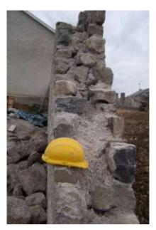
The final picture shows a cross section of a stone wall under construction. The space between the two faces of the wall is filled with mortar. When the wall is finished, this mortar will not be seen.
