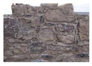
You can see a line which the men have stretched to mark a horizontal level on the wall, so that the stones can be laid in courses. This gives a coursed rubble wall. In the top courses, the mortar can still be seen on the surface of the stone, but lower down the joints have been pointed, so that the stones seem to stand out a bit.
