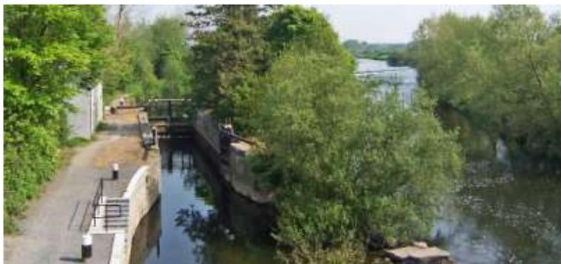
This lock is on the River Barrow at Leighlinbridge. The main river channel is on the right and upriver you can see the weir which diverts some of the flow of the river into a short canal. There are two pairs of lock gates. The upper gates are closed and
